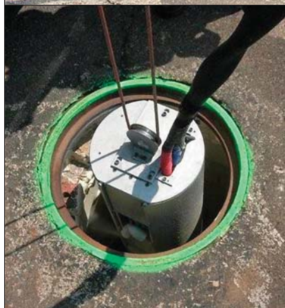
Above, ROI president Mike Kronz deploys the spray unit to start the sealing process. At left, the sprayer unit is deployed down the manhole.
