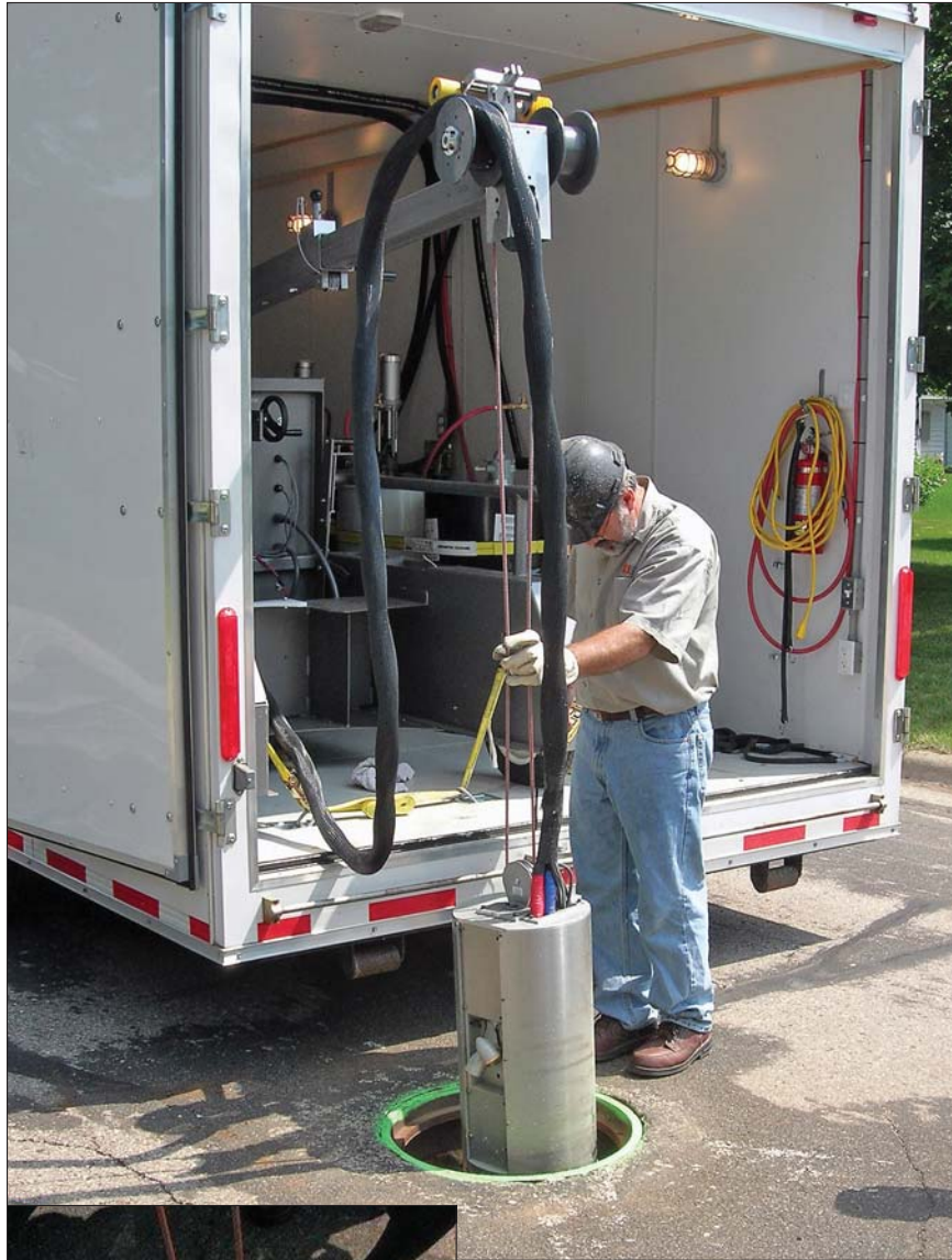
Above, ROI president Mike Kronz deploys the spray unit to start the sealing process. At left, the sprayer unit is deployed down the manhole.
